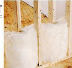
Staggered Wall Studs
